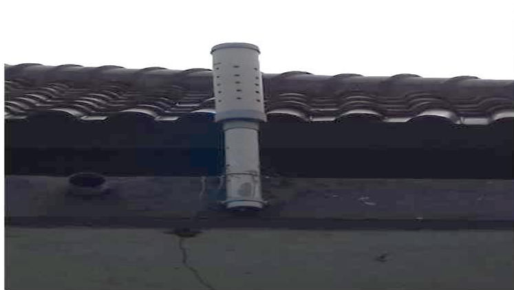
Gambar 46. Lightning Detector bertipe LD-250
